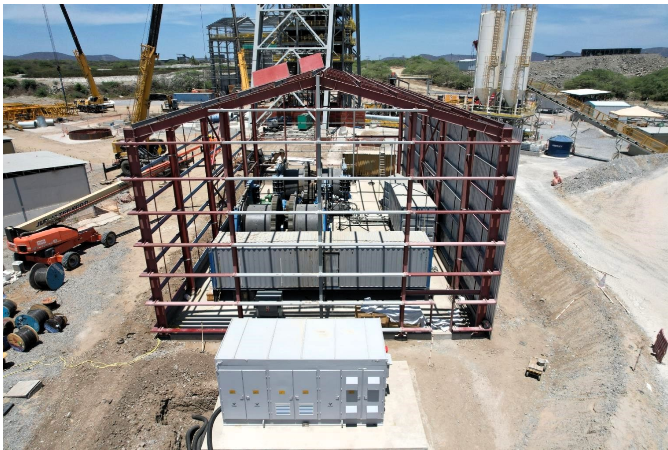
Figure 3: Progress on erection of the stage winder building (October 2023).
