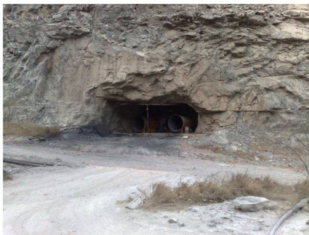
Figure 18-22: Old pit exhaust fans – model TECSIS (MCSA, 2020)
