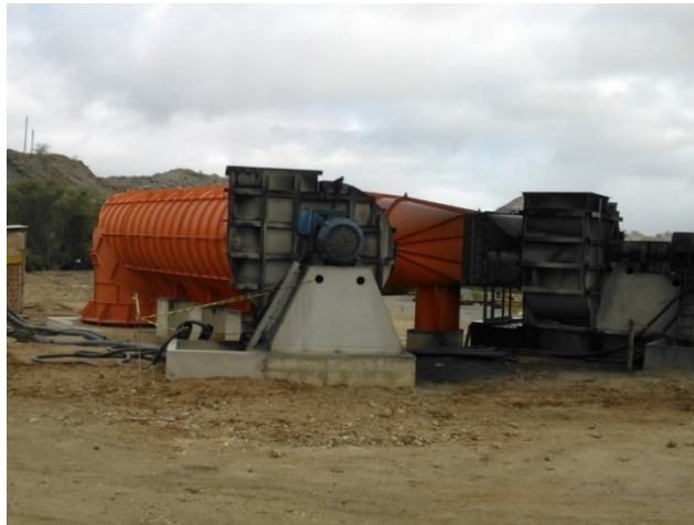
Figure 18-21: P1/P2 exhaust fans – model SOMAX (MCSA, 2020)
