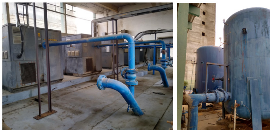
Figure 18-16: Compressed air central station and pressure vessels at surface (MCSA, 2020)
