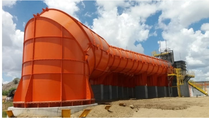
Figure 18-20: P3 exhaust fans – model SOMAX (MCSA, 2020)
