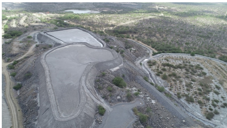
Figure 20-6: Photograph of Co-disposal Method on completion of Deposition (MCSA, 2019)
