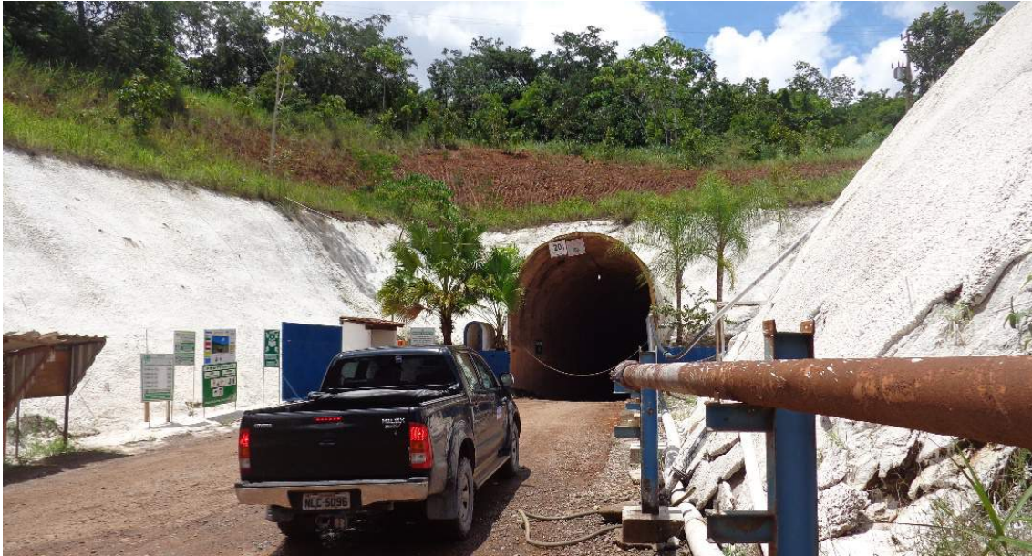
Figure 4. Mine Portal (NX Gold, 2018)
