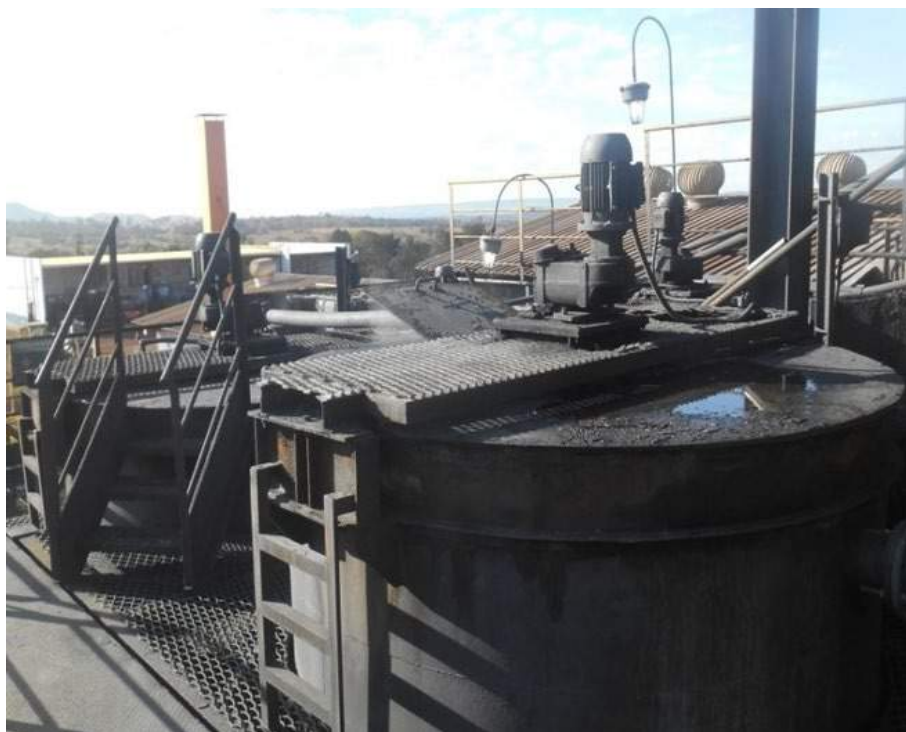
Figure 73. CIL (Carbon-in-leach) Unit overview.
