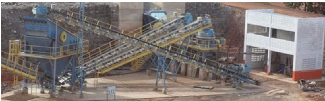
Figure 68. Crushing Unit overview.
