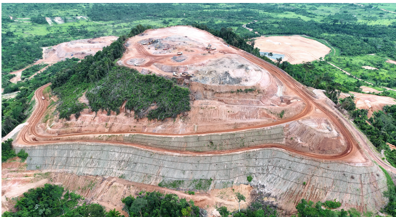
Figure 1: Tucumã Project pre-stripping progress (February 2023).
