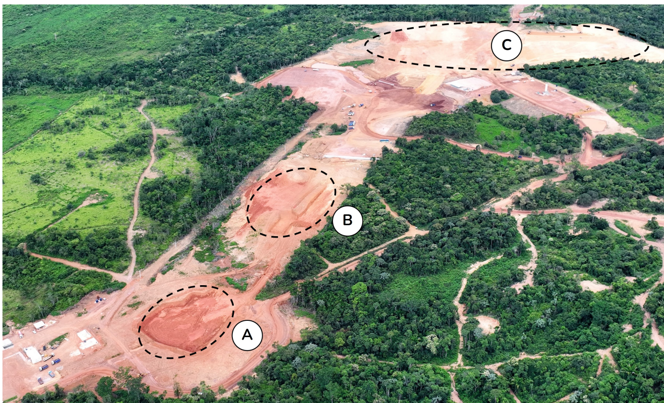
Figure 2: Aerial view of future Tucumã Project processing areas, including (A) primary crushing, (B) secondary and tertiary crushing, and (C) plant and administrative buildings.
