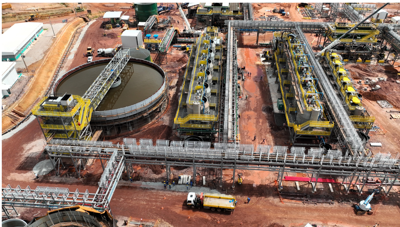
Figure 1: The Tucumã Project's flotation circuit and tailings thickener (May 2024).
