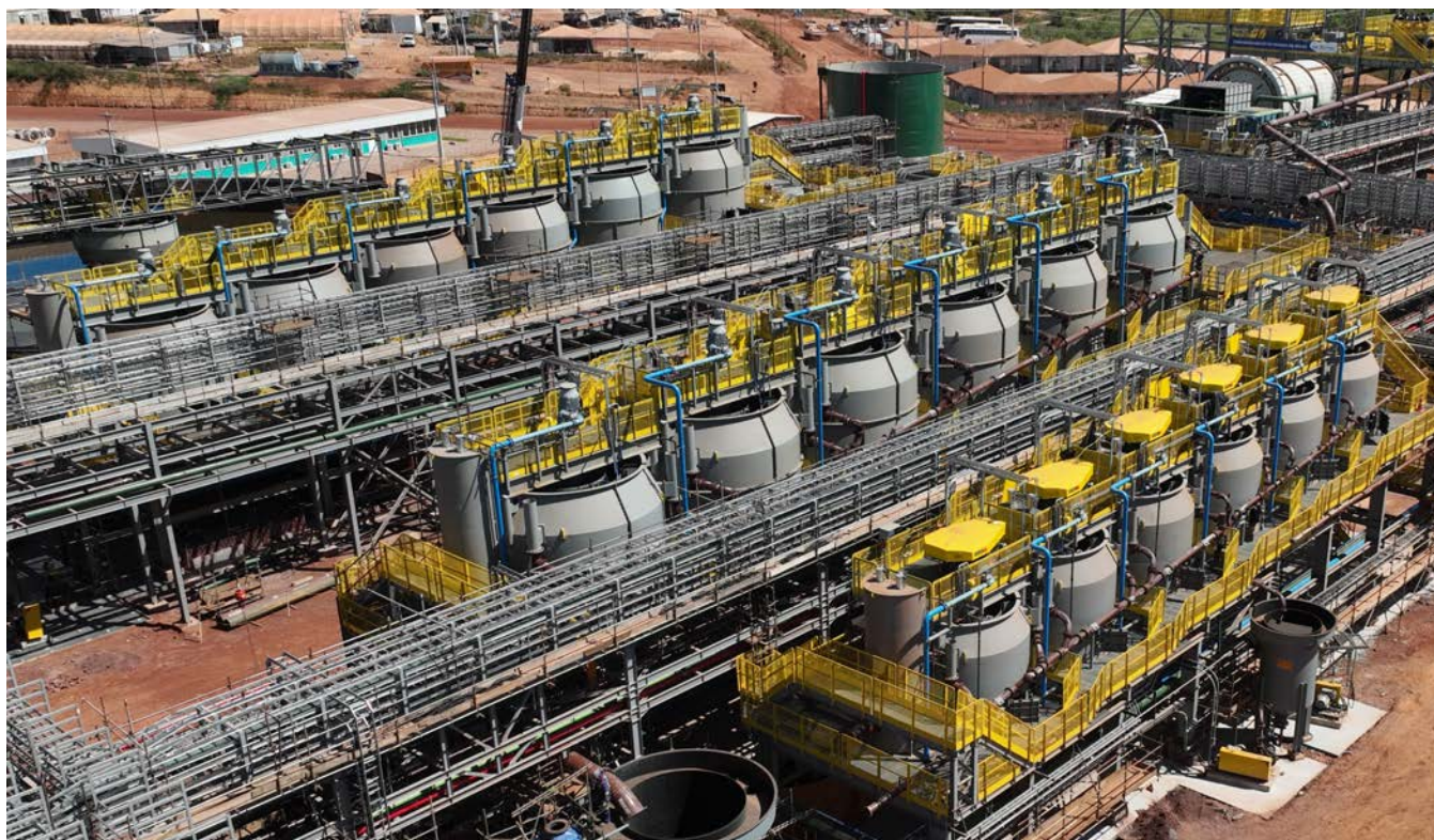
Figure 5: Completion and commissioning of flotation circuit as of June 2024.
