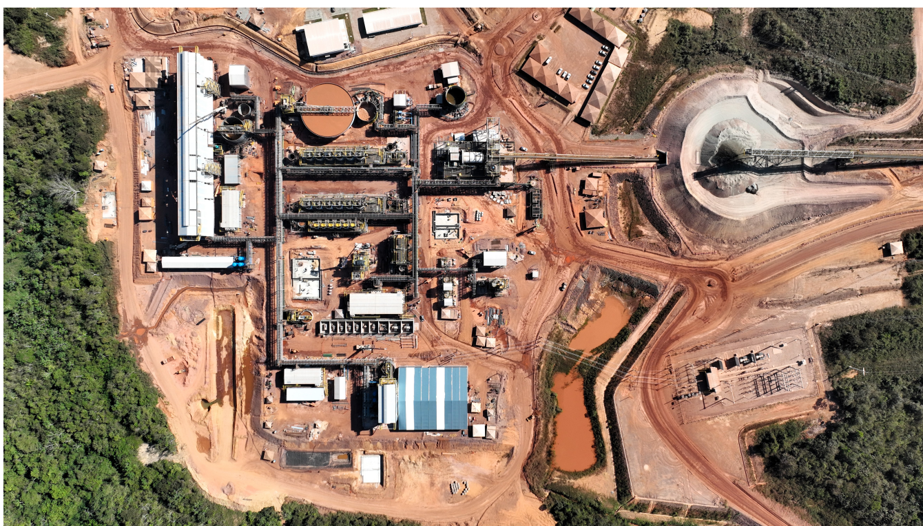
Figure 2: Aerial view of the Tucumã Project's process plant, including ball mill, flotation and filtration (center), concentrate shed (bottom), and crushed ore stockpile (right) (July 2024).
