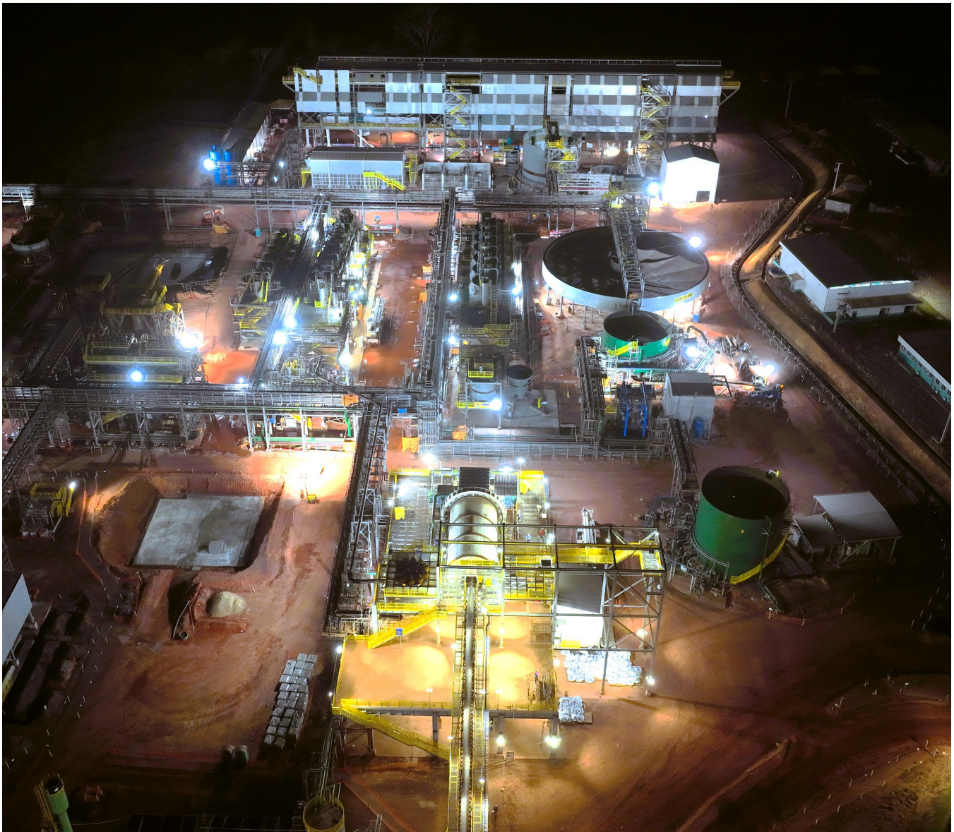
Figure 3: Night-time aerial view of the Tucumã Project's process plant, including ball mill, flotation and filtration, taken during the first 24-hour shift of continuous mill operations (July 2024).
